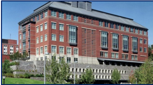
CUE Public Parking Garage
