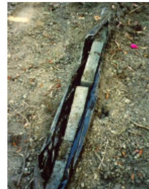
**Figure 7** Root barriers made of unit pavers wrapped in plastic.
