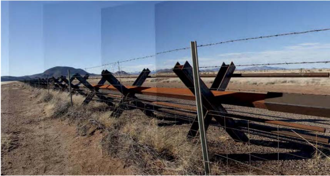
Vehicle barriers along the US-Mexico border. From: "Continental Divide: Wildlife, People, and the Border Wall"
