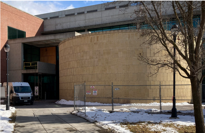
The drum prior to demo.
