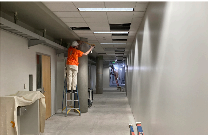
Paint prep of the cable trays.
