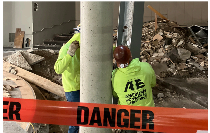
American Ironworks & Erectors installing the new steel columns.
