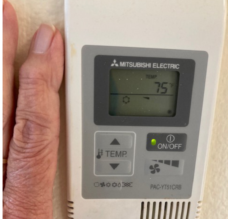
Photo for scale of a thermostat's small buttons and indicators, which are difficult for senior living residents to understand and interact with.
