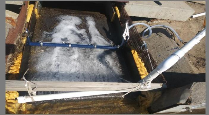
In the picture above I worked with the irrigation specialist to create a new screen in the water drop as well as adding pressurized water to help self-clean with the use of pvc pipes, tubing, and spray nozzles and clamps.
