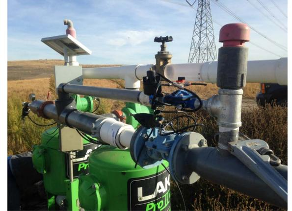
This is a sand media filter station that I designed and built. It has two pressure control valves. A 3 inch valve and an inch and a half valve. I designed it with two valves so that we could water the entire 40 acre vineyard at once if desired, or we can water individual blocks or sub blocks as small as one and a half acres.
