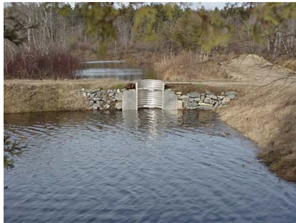
Flume with riprap
