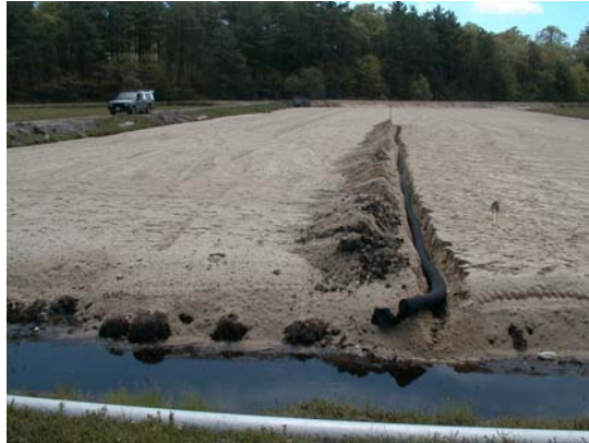
Installation of a drainage pipe on a newly prepared farm surface
