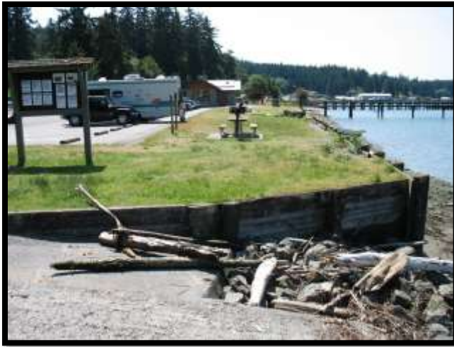
Figures 6-7: Hard shoreline armor is removed and regraded to protect and stabilize the shoreline. Cornet Bay on Whidbey Island. Image Credit: Sarah Schmidt
