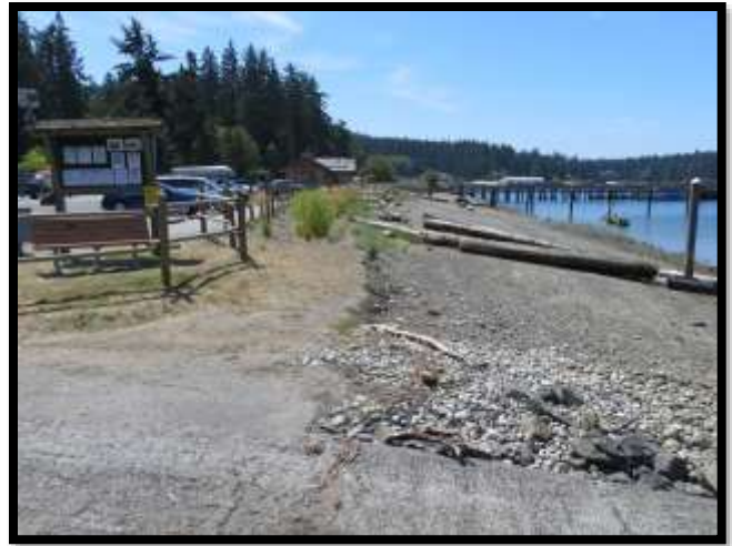
Figures 6-7: Hard shoreline armor is removed and regraded to protect and stabilize the shoreline. Cornet Bay on Whidbey Island. Image Credit: Sarah Schmidt
