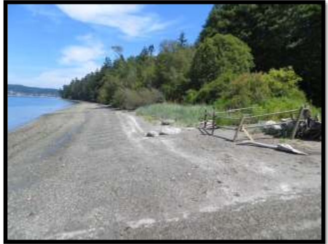
Figures 4-5: Hard shoreline armor is removed and regraded with sand and gravel to match the natural beach slope. Cornet Bay on Whidbey Island. Image Credit: Sarah Schmidt
