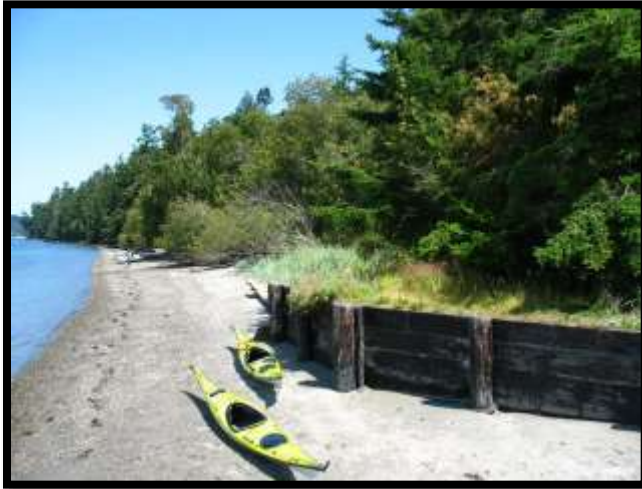
Figures 4-5: Hard shoreline armor is removed and regraded with sand and gravel to match the natural beach slope. Cornet Bay on Whidbey Island. Image Credit: Sarah Schmidt
