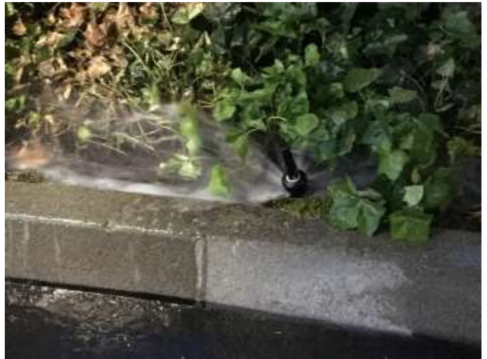
Figure 6: Make sure to monitor your irrigation systems periodically for any maintenance issues and to ensure that the intended amount of water is reaching the right plants and not ending up on paved areas. Image Credit: Jerilyn Ritzman.
