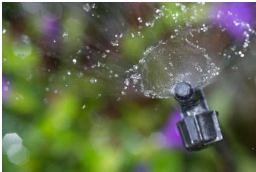
Figure 1: Refining irrigation practices can help conserve water during dry summers and droughts, but it's just one of seven principles of xeriscaping that can help create a long-term waterwise landscape. Image Credit: Oregon State University / CC BY-SA 2.0 . Wikimedia Commons (link) .
