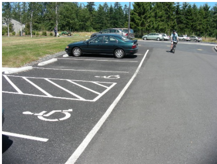
Photo at left: porous asphalt used for parking stalls on sloped entry road at Breazeale Interpretive Center, Padilla Bay National Estuarine Research Reserve, Skagit County:
