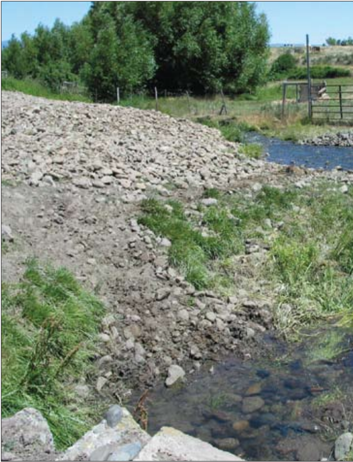
Figure 6. Hardened water access area (Photo by Tipton Hudson)
