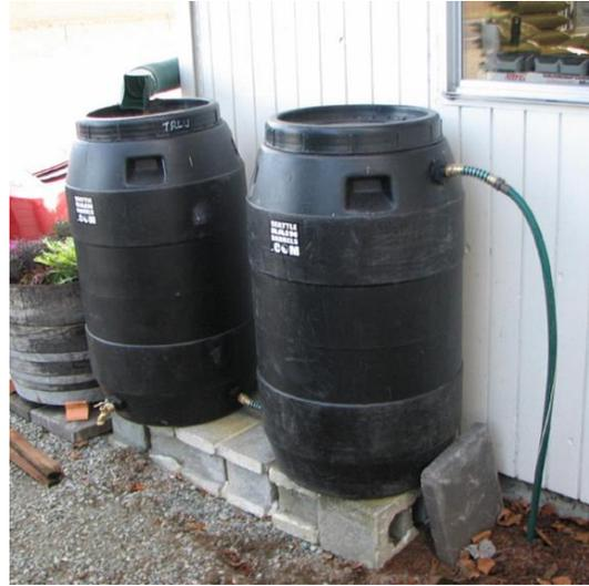
**Left:** Downspout flowing directly into a rain barrel with a mesh guard on top to keep debris and mosquitoes out of the barrel. **Right:** Rain barrels connected at the base (note that overflow pipe should be directed to a safe place for any excess water to disperse). *Photos are with permission from Gardener's Supply Company.*
