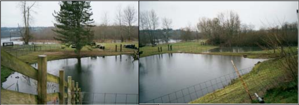
Pond drains to surface water
