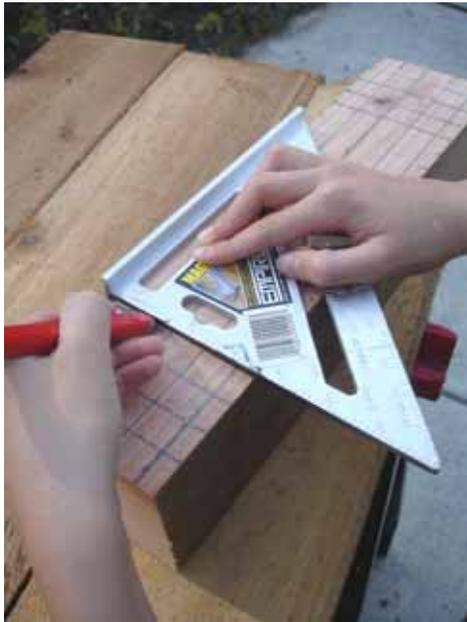
Choose a 4x4 or 4x6 block of pine or fir (*not* treated wood). Cut a slight downward angle on one end to give the roof a little slope. Draw a grid of lines  $\frac{3}{4}$ -inch apart on the “downward slope” side of the block (the shorter side). Photo by Jason Miller
