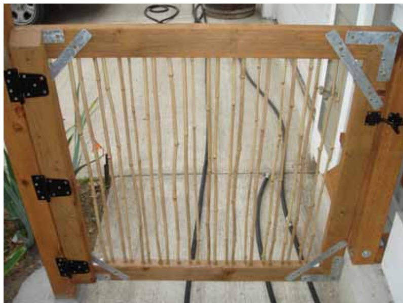
Plenty of bracing helps to ensure this gate will never sag. Note the hinges, which are placed on the back side of the gate to allow an inward swing. Photo by Jason Miller
