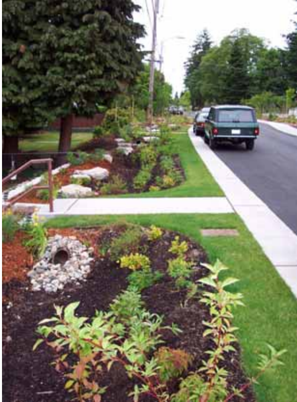
Rain gardens can be shaped and sized to fit almost any space, even the sometimes problematic boulevard areas bordering streets. Photo by Seattle Public Utilities
