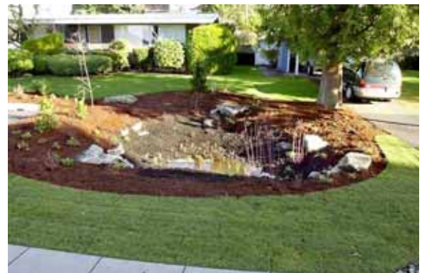
A newly planted rain garden in Seattle. Rain gardens are one of the most versatile and effective tools in a new approach to managing storm water called low impact development (LID). Photo by Seattle Public Utilities
