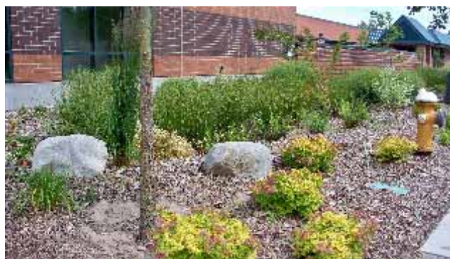
Above: Skagit Conservation District and Skagit Backyard Wildlife members installed this rain garden following plans by Eccos Designer LLC in 2010 for the Skagit County Commissioners building on Continental Place in Mount Vernon. The garden filters water from the building's roof. Below: The commissioner's rain garden is shown thriving in summer 2010. Photos courtesy of Skagit Conservation District.
