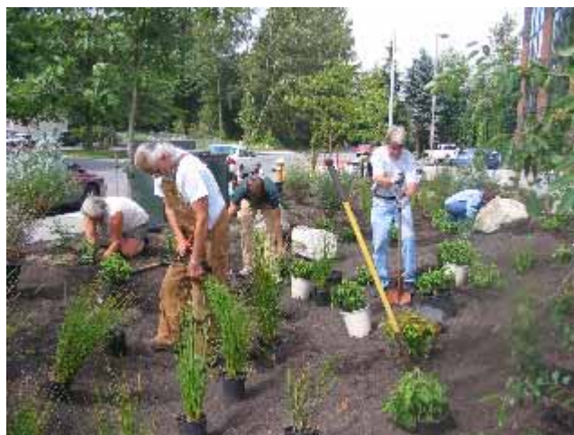
Above: Skagit Conservation District and Skagit Backyard Wildlife members installed this rain garden following plans by Eccos Designer LLC in 2010 for the Skagit County Commissioners building on Continental Place in Mount Vernon. The garden filters water from the building's roof. Below: The commissioner's rain garden is shown thriving in summer 2010. Photos courtesy of Skagit Conservation District.
