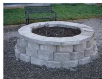
A raised bed made with concrete blocks
