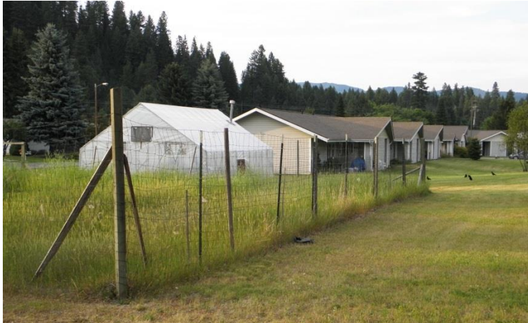
LOOKING NORTH AT ABANDONED GARDEN AND GREENHOUSE WITH QUAIL MANOR (SUBSIDIZED HOUSING FOR DEVELOPMENTALLY DISABLED ADULTS) IN BACKGROUND.
