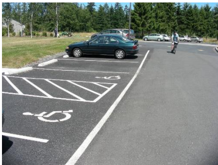
Photo at left: porous asphalt used for parking stalls on sloped entry road at Breazeale Interpretive Center, Padilla Bay National Estuarine Research Reserve, Skagit County: http://www.ecy.wa.gov/programs/sea/padillabay/index.html Photo by Scott Chase
