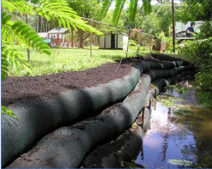
Bio-filter wattles filled with compost
