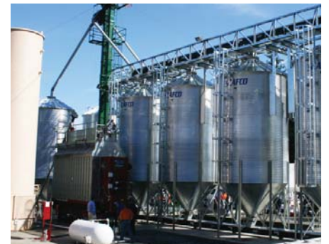
Snohomish County's seed dryer and storage facility at Cathcart
