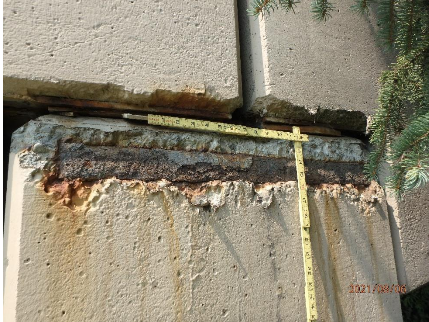
Photo 71: Spall in East Face of Pier 3 Cap, Looking West
