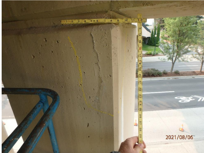
Photo 91: Delamination in Top Northwest Corner of Pier 2B, Looking South
