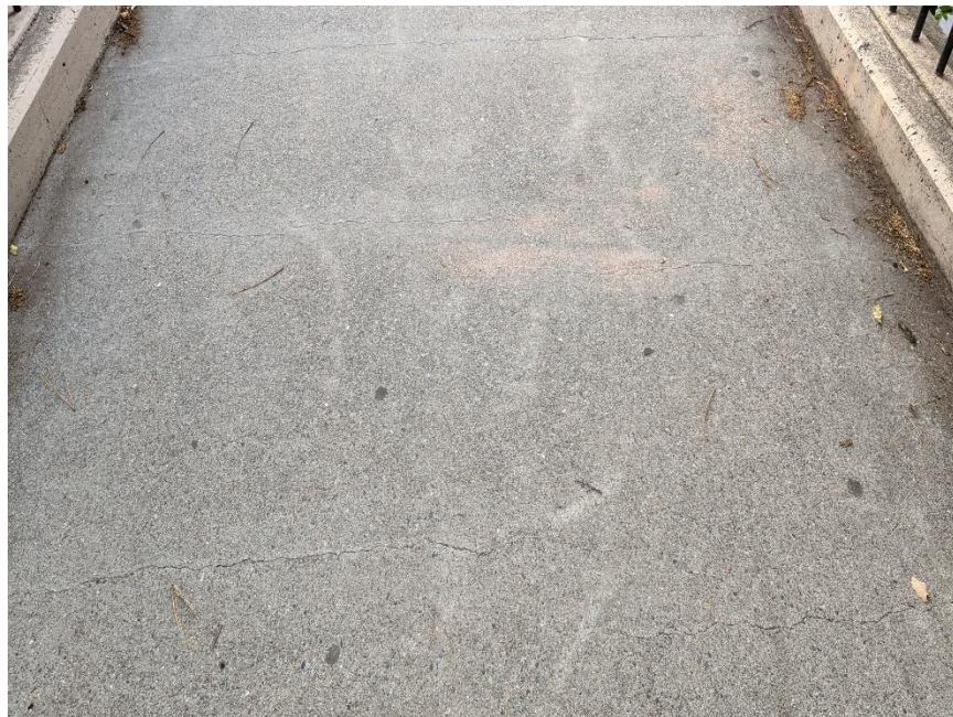
Photo 14: Typical Transverse Cracking in Top of Deck, Looking South
