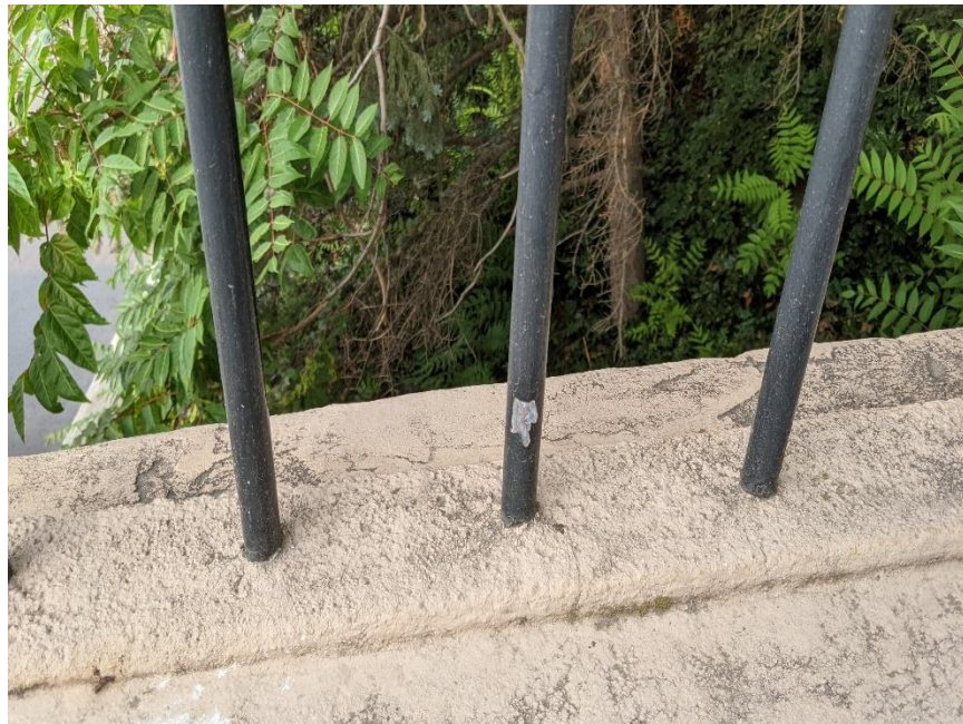
Photo 78: Typical Minor Impact Damage and Chipped Paint in Metal Rail
