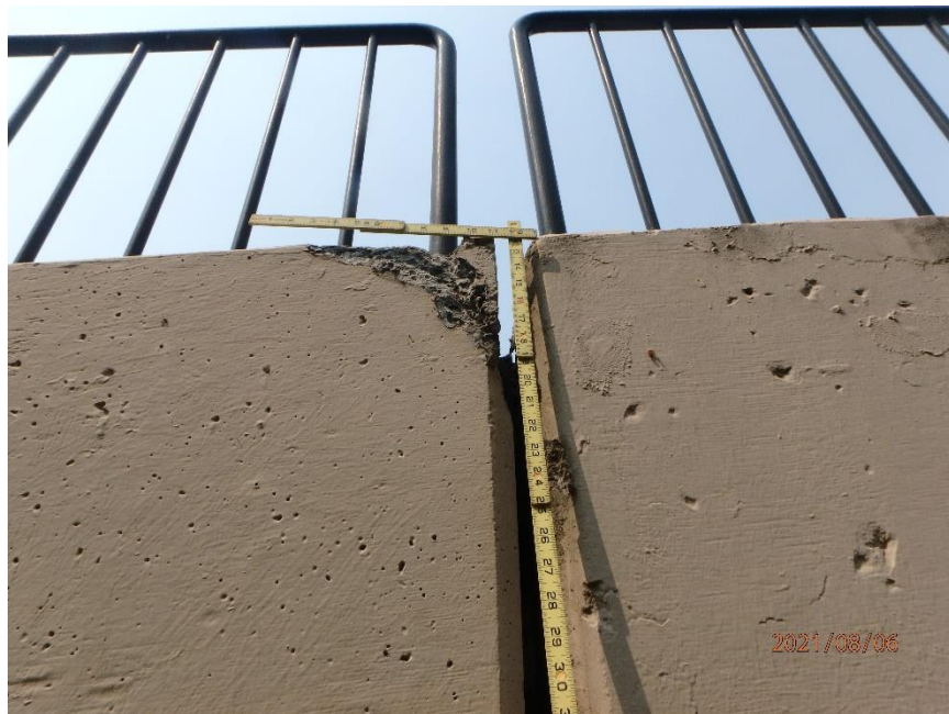
Photo 28: Spall in East Face of Span 1 East Girder at Top Corner at North End, Looking West
