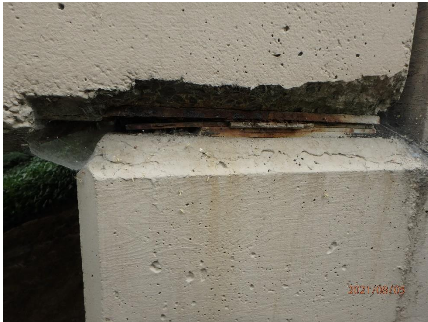
Photo 50: Spall in Span 4 East Girder on the East Face at the North End above the bearing plate, Looking West
