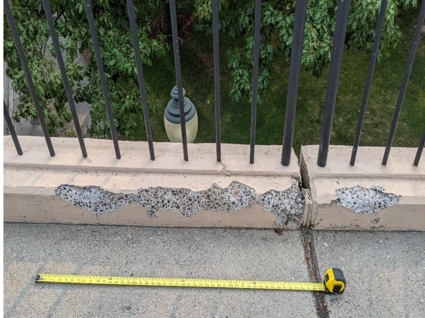
Photo 81: 4FT Long Spall in Span 3 East Curb at South End, Looking East
