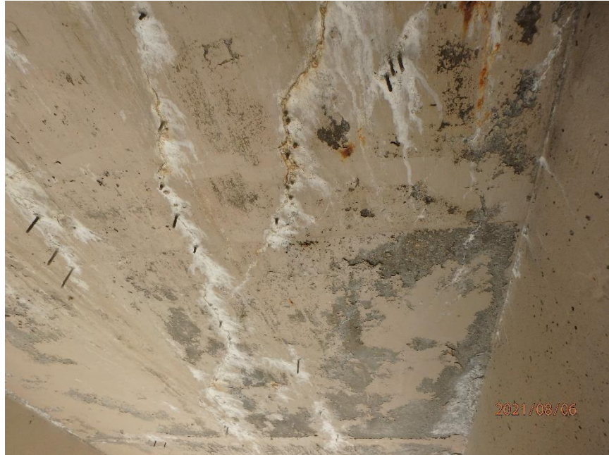
Photo 21: Longitudinal Cracking at Pier 2 Underdeck, Looking South
