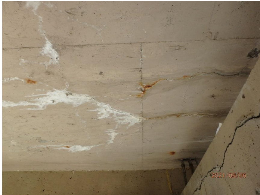
Photo 20: Typical Longitudinal Cracking in the Underdeck, Looking East
