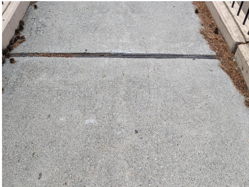
Photo 84: Typical Expansion Joint, Looking South
