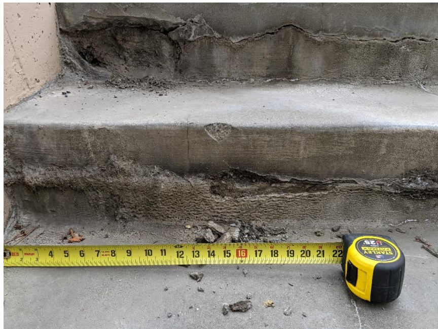
Photo 88: Cracks in Bottom Two Stairs, Looking South
