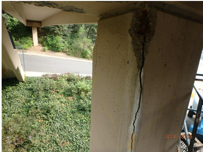
Photo 60: Delamination in Pier 2, Looking Northeast
