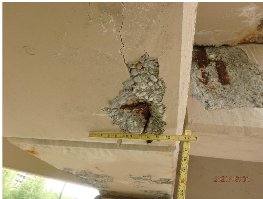
Photo 93: Spall in Underside of Pier 2B Cap at East End, Looking East
