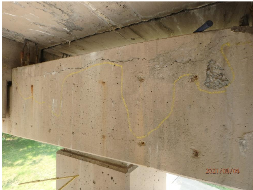
Photo 54: Delamination of the North Face of Pier 1 Cap, Looking Southeast (Yellow Lines Show Delamination)
