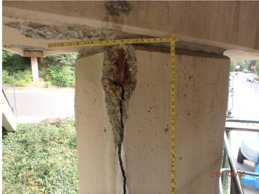
Photo 63: Spall in Southwest Corner of Pier 2, Looking Northeast
