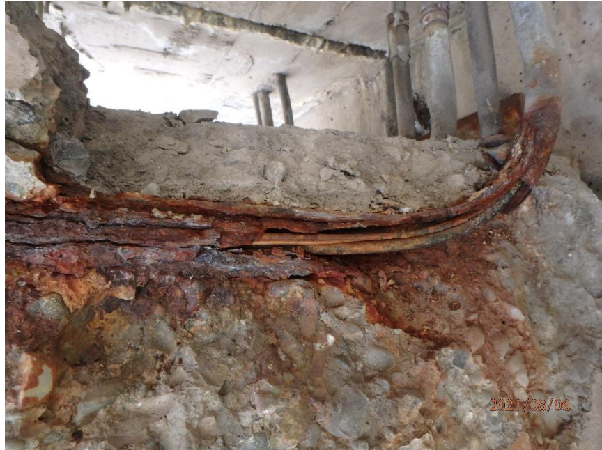
Photo 57: Exposed Wire and Corroded Steel Conduit at Pier 1 Cap, Looking North
