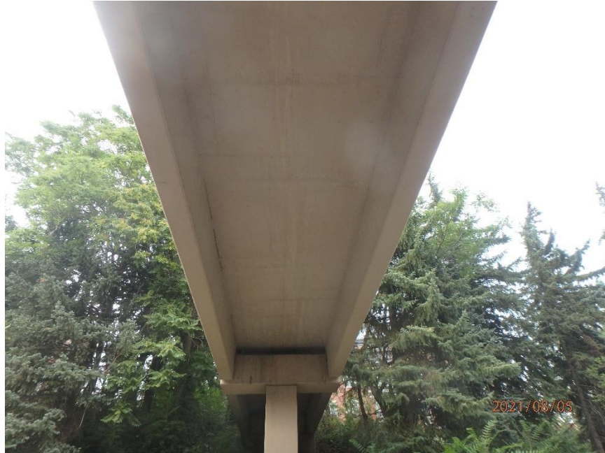
Photo 17: Typical Transverse Cracking in the Underdeck, Looking North
