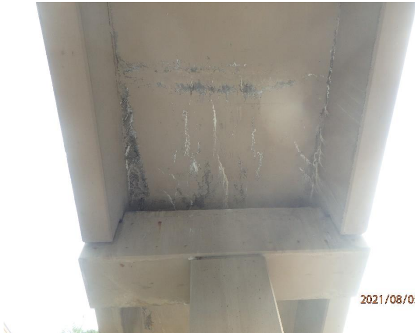
Photo 18: Typical Longitudinal Cracking in the Underdeck, Looking South
