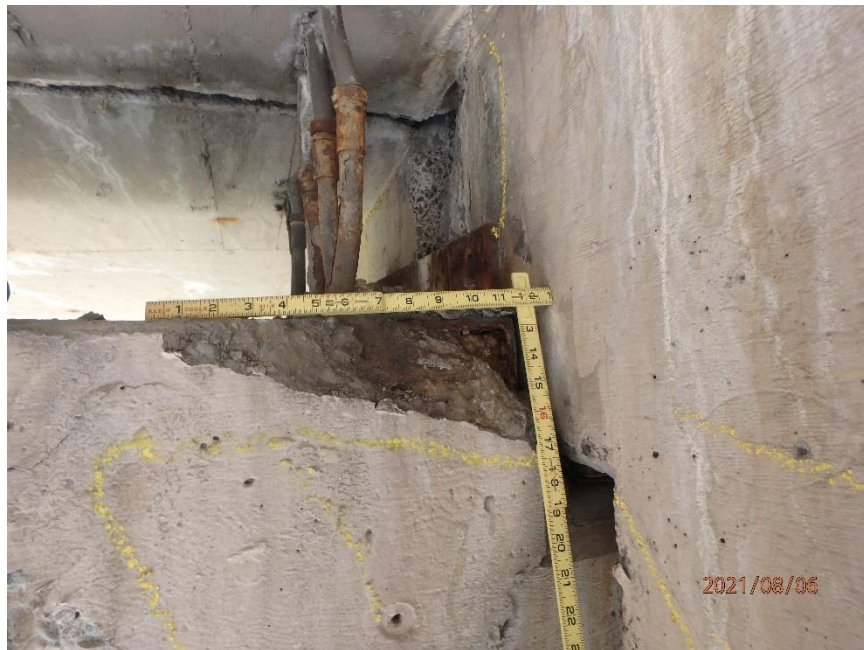
Photo 58: Spall in West Top Corner of Pier 1 Cap North Face, Looking South
