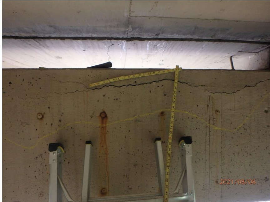
Photo 69: Delamination of the North Face of Pier 3 Cap Top Corner, Looking South
