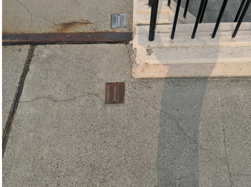
Photo 13: Typical Cracking Around Snow Melt Junction Boxes, Looking West
