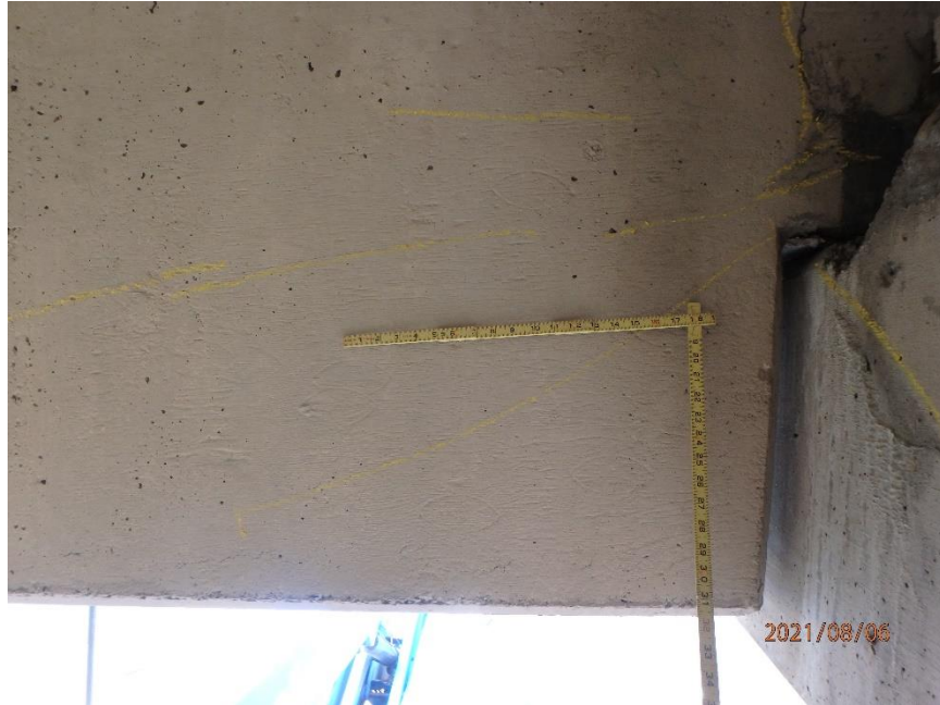
Photo 27: Diagonal Cracks in East Face of Span 1 West Girder at North End, Looking West
