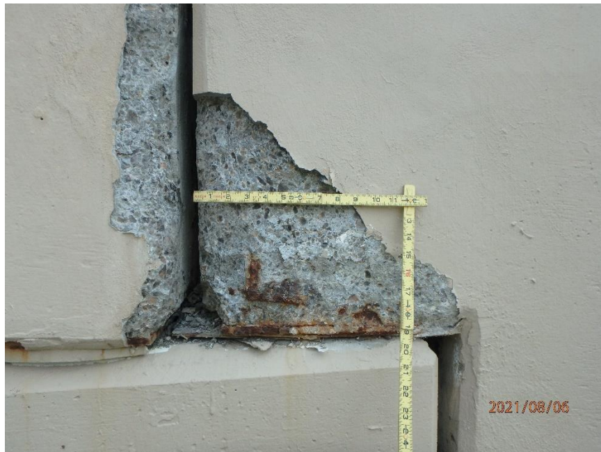
Photo 30: Spall in West Face of Span 1 West Girder at bottom edge at North End. Looking East
