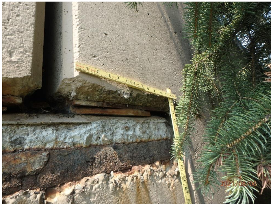
Photo 48: Spall in Span 4 East Girder on the East Face at the South End, Looking Northwest
