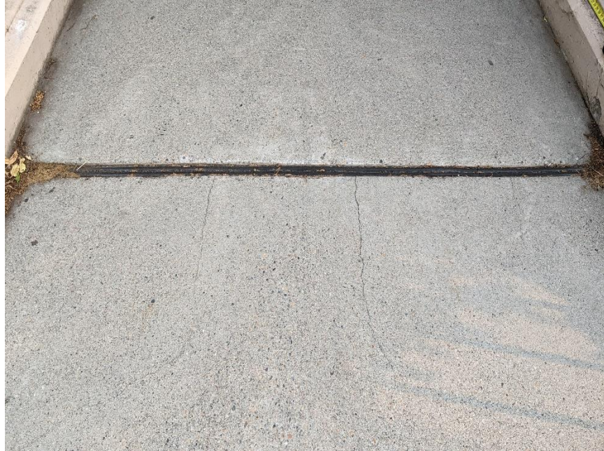
Photo 83: Typical Expansion Joint, Looking North
