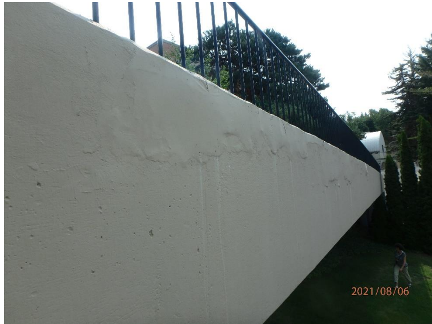
Photo 25: Typical Unsound Patches in West Face of west Girder Top Edge, Looking Southeast
