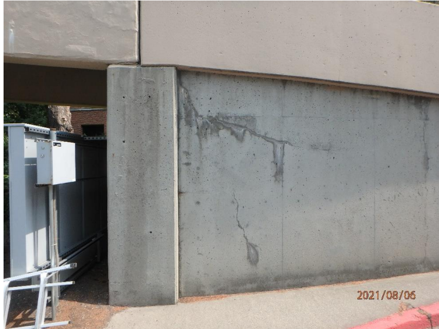
Photo 51: Hairline Cracks with Light Efflorescence in South Abutment West Side, Looking East
