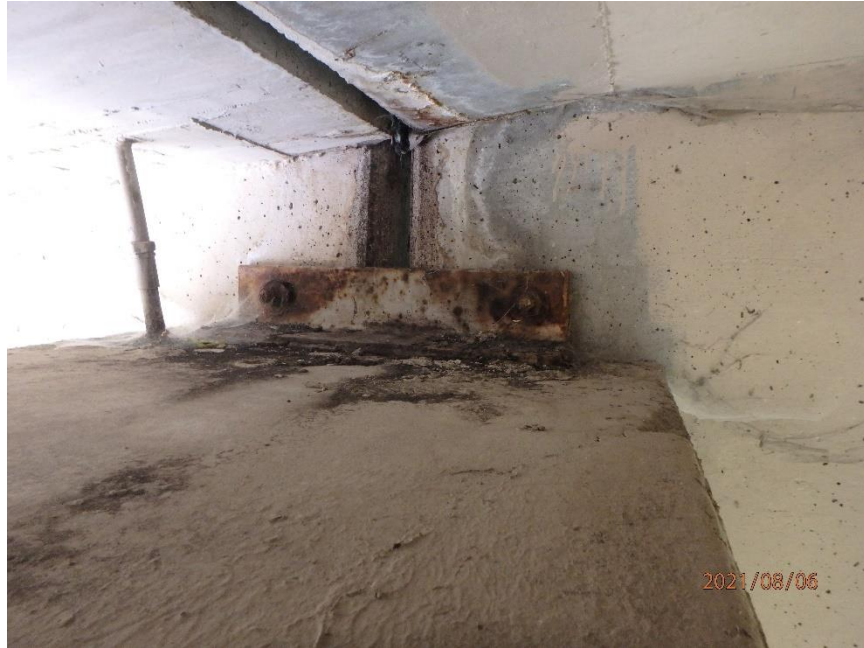
Photo 35: Typical Steel Connection Bracket at Pier Caps, Looking West
