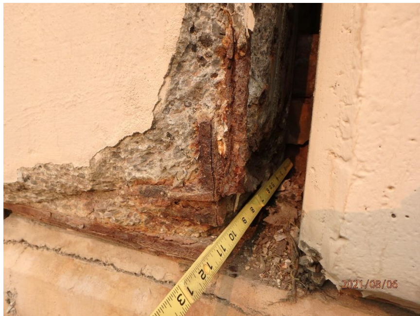
Photo 40: Spall in Span 2 East Girder at Northeast corner, Looking Southwest
