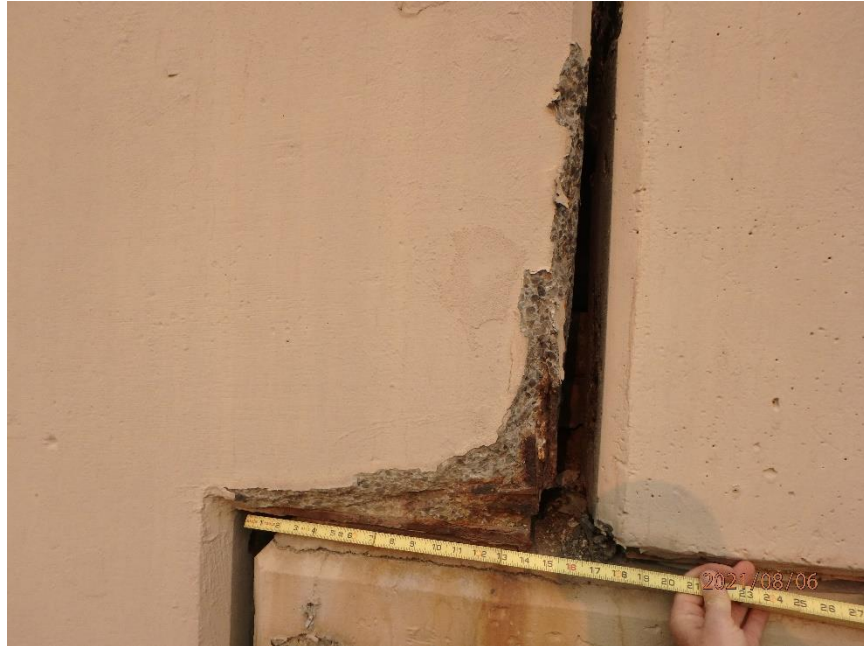
Photo 39: Spall in Span 2 East Girder at Northeast corner, Looking West
