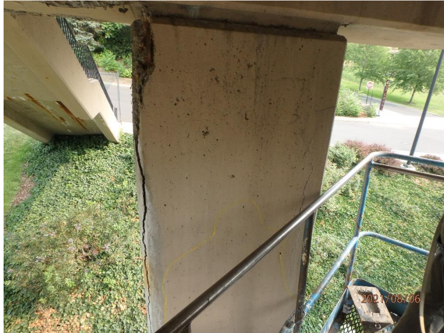
Photo 59: Delamination in Pier 2, Looking North
