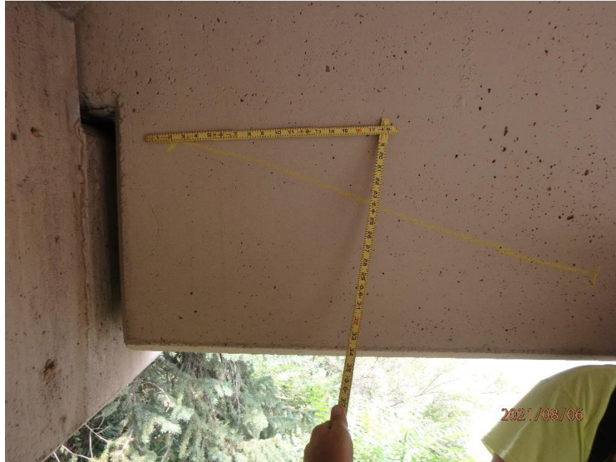
Photo 47: Diagonal Cracks in West Face of Span 3 East Girder at North End, Looking East
