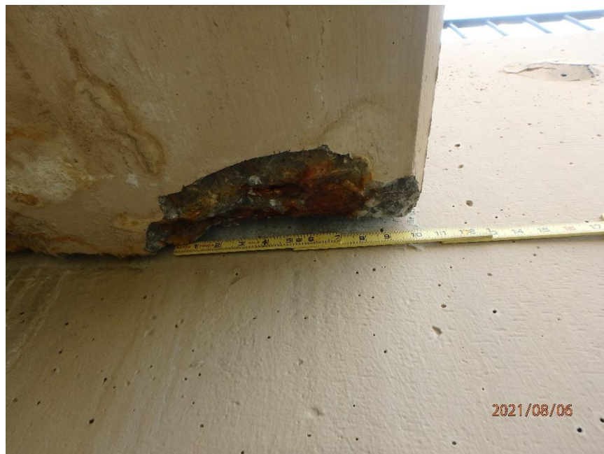
Photo 96: Spall in Southeast Bottom Corner of South Stair Girder, Looking East
