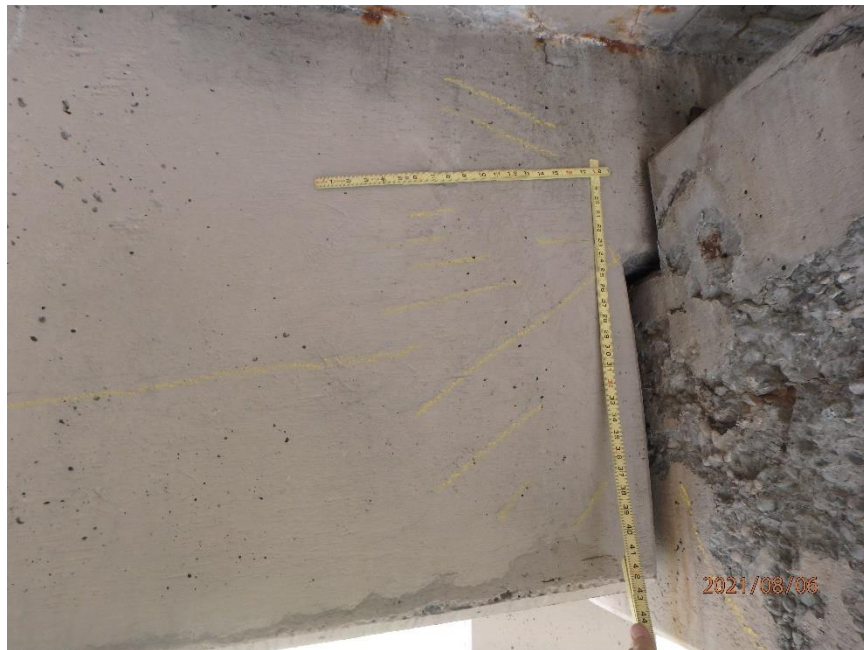
Photo 38: Diagonal Cracks in East Face of Span 2 West Girder at North End, Looking West
