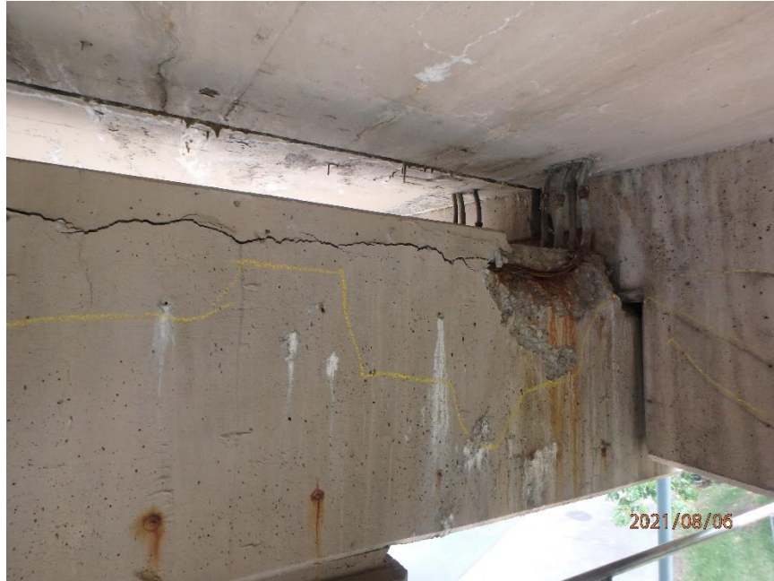
Photo 53: Delamination of the South Face of Pier 1 Cap, Looking Northeast (Yellow Lines Show Delamination)
