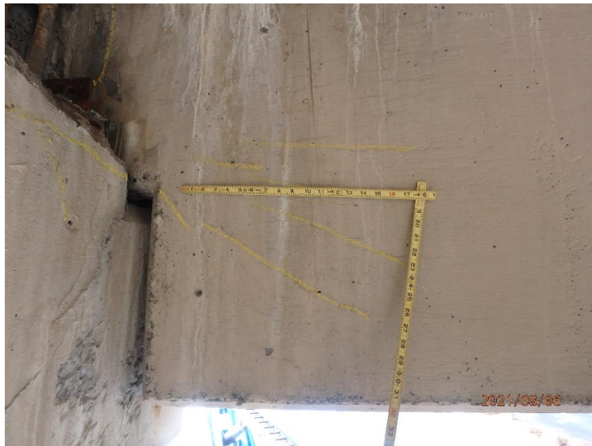
Photo 32: Diagonal Cracks in East Face of Span 2 West Girder at South End, Looking West
