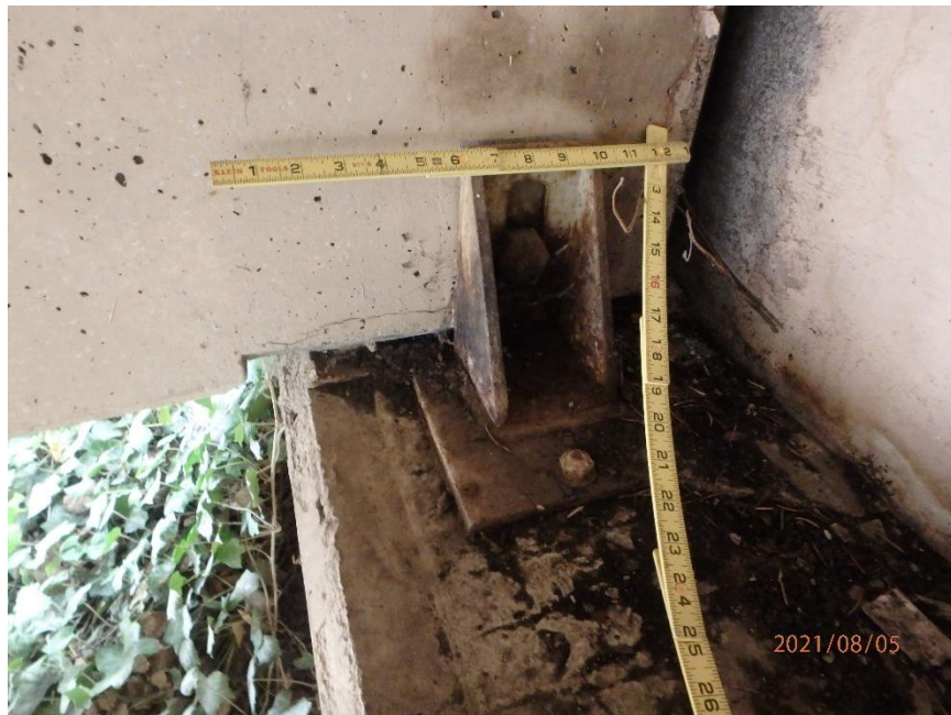
Photo 34: Typical North Abutment Steel Connection Bracket, Looking West
