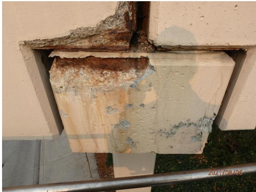
Photo 64: Spall and Scaling in East Face of the Pier 2 Cap, Looking West
