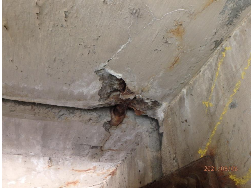
Photo 23: Spall in Southwest Corner of Span 3 Underdeck Above Pier 2, Looking Southwest
