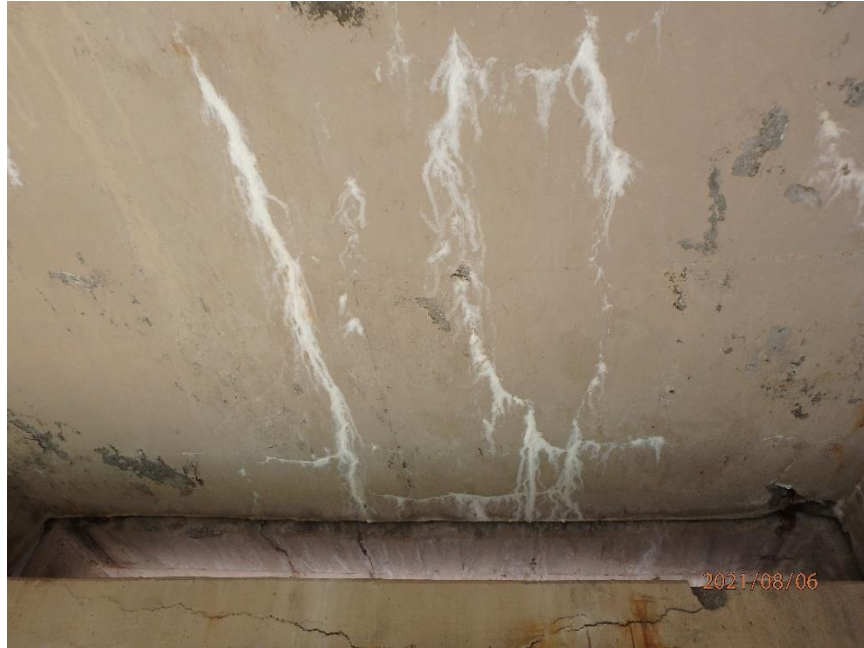
Photo 19: Typical Longitudinal Cracking in the Underdeck, Looking South
