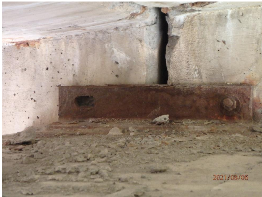
Photo 42: Sheared off Bolt at Pier 2 Connection Hardware, Looking West
