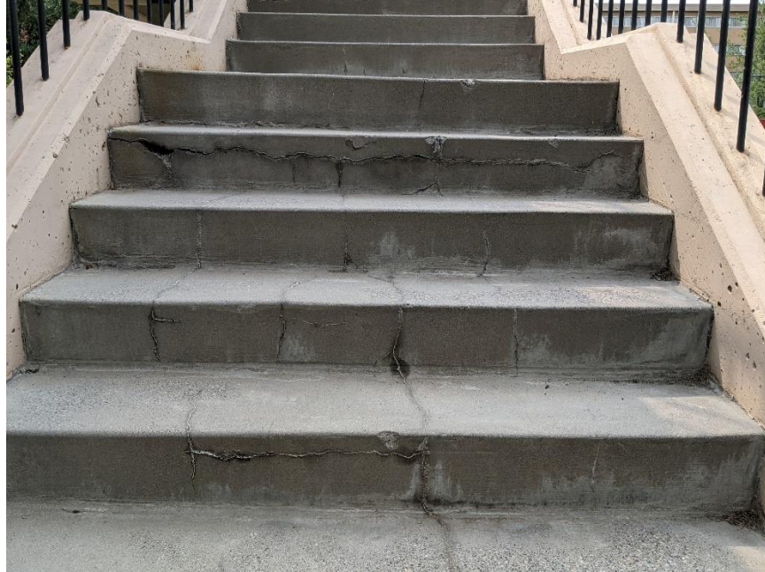
Photo 85: Typical Cracking in Stair Treads and Risers, Looking South
