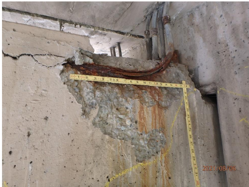
Photo 56: Spall in East Top Corner of Pier 1 Cap South Face, Looking North
