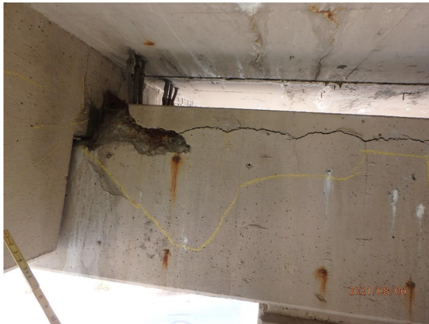
Photo 52: Delamination of the South Face of Pier 1 Cap, Looking Northwest (Yellow Lines Show Delamination)
