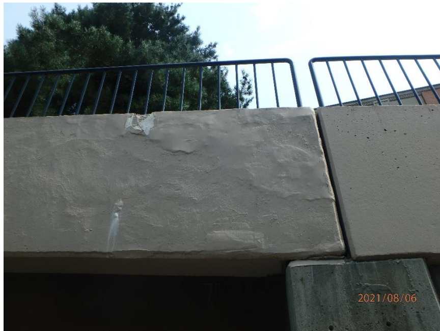
Photo 24: Typical Unsound Patches in West Face of West Girder, Looking East
