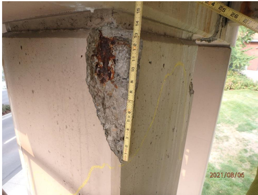
Photo 61: Spall in Northeast Corner of Pier 2, Looking Southwest
