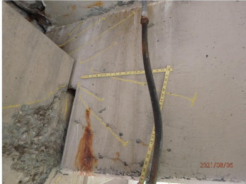
Photo 45: Diagonal Cracks in East Face of Span 3 West Girder at South End, Looking West
