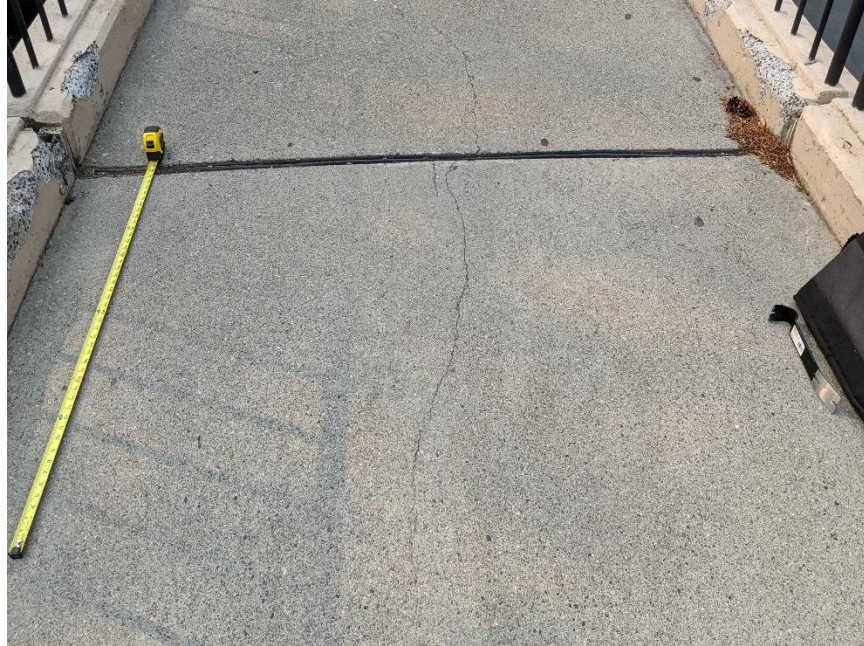
Photo 15: Typical Longitudinal Cracking from Deck Joints in Top of Deck, Looking North
