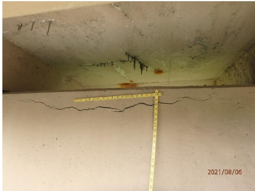
Photo 93: Delamination and Cracking of the South Face of Pier 2B Cap Top Corner, Looking North
