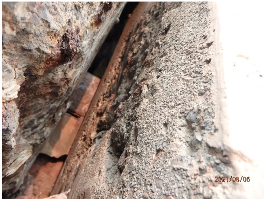
Photo 46: Spall in South Face of East Girder at South End, Looking Northwest
