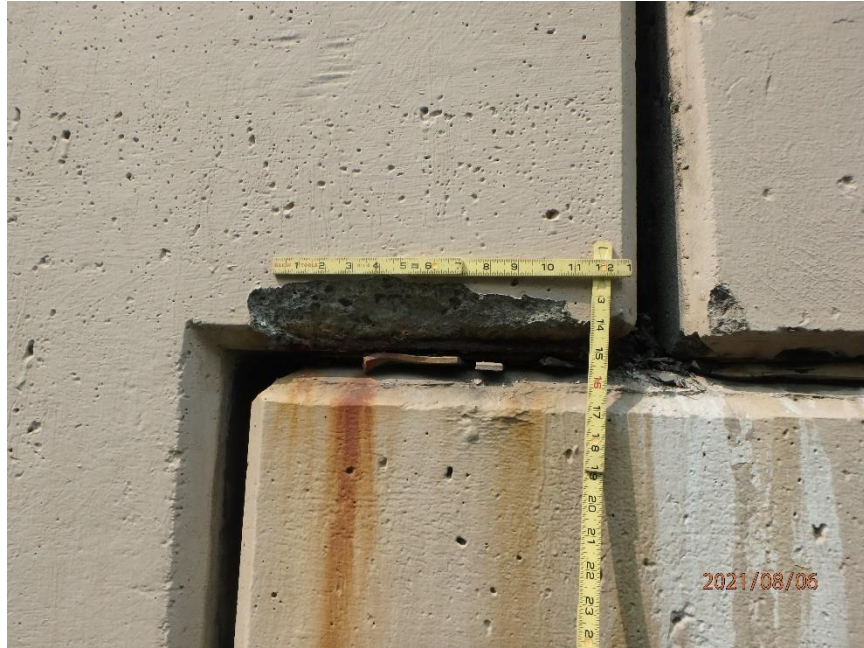
Photo 29: Spall in East Face of Span 1 East Girder at bottom edge at North End. Looking West
