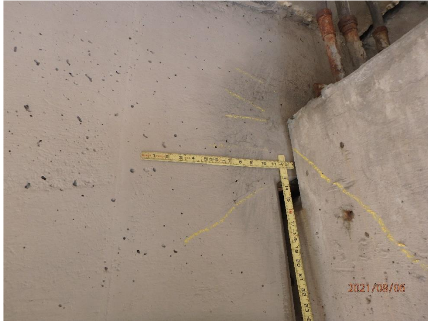
Photo 31: Diagonal Cracks in West Face of Span 2 East Girder at South End, Looking East
