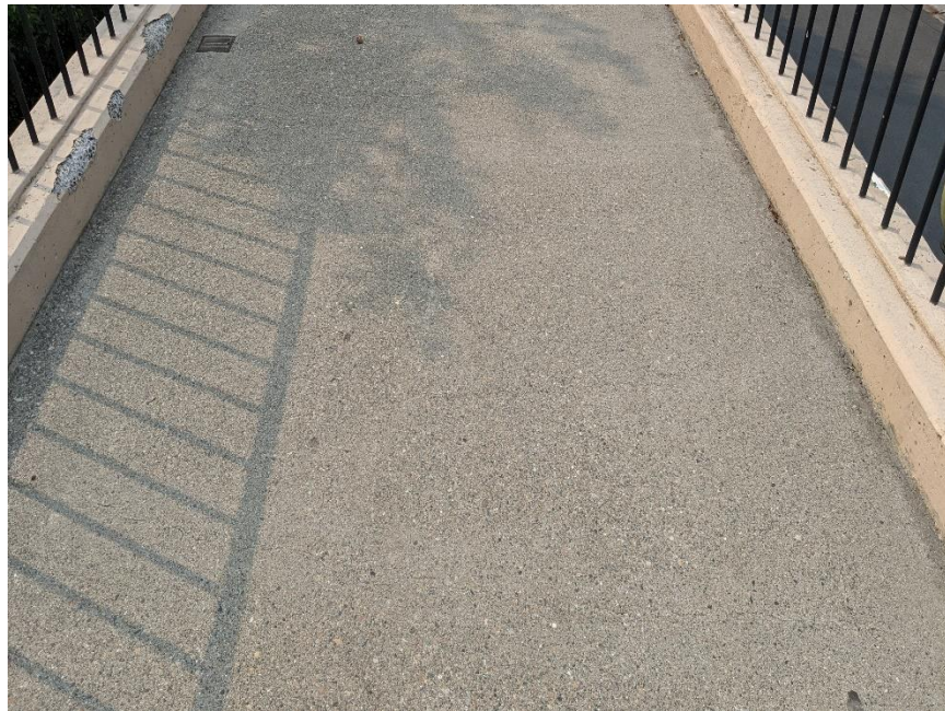
Photo 12: Typical Minor Scaling in Top of Deck, Looking South
