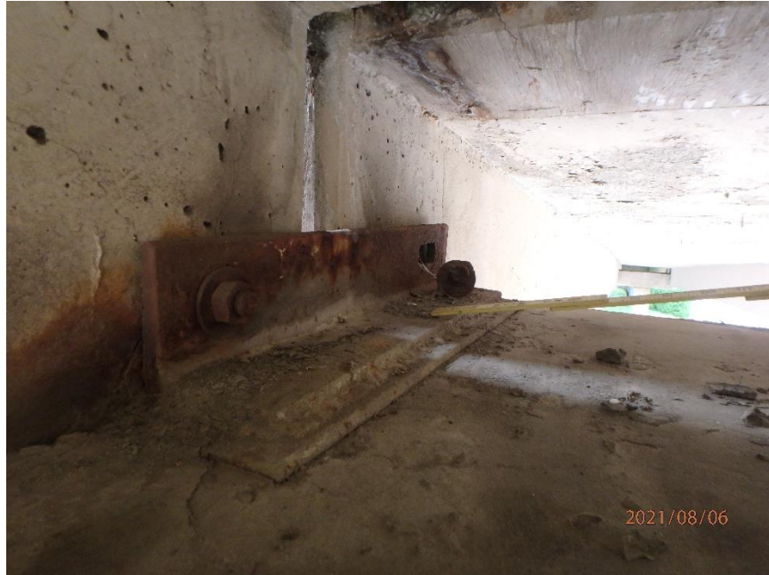
Photo 43: Sheared off Bolt at Pier 2 Connection Hardware, Looking Southeast
