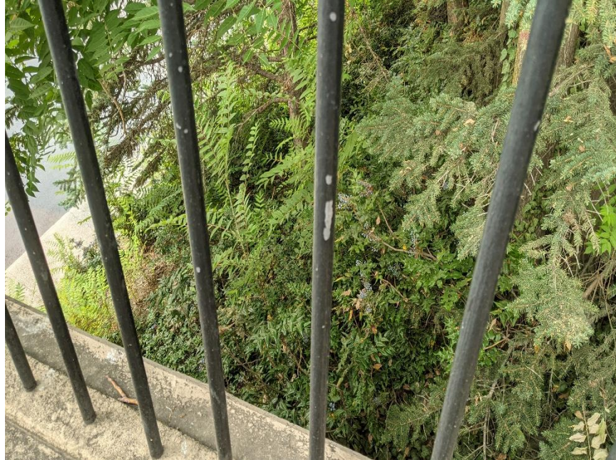
Photo 77: Typical Minor Impact Damage and Chipped Paint in Metal Rail
