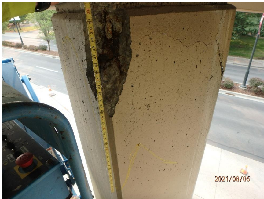
Photo 62: Spall in Northwest Corner of Pier 2, Looking Southeast
