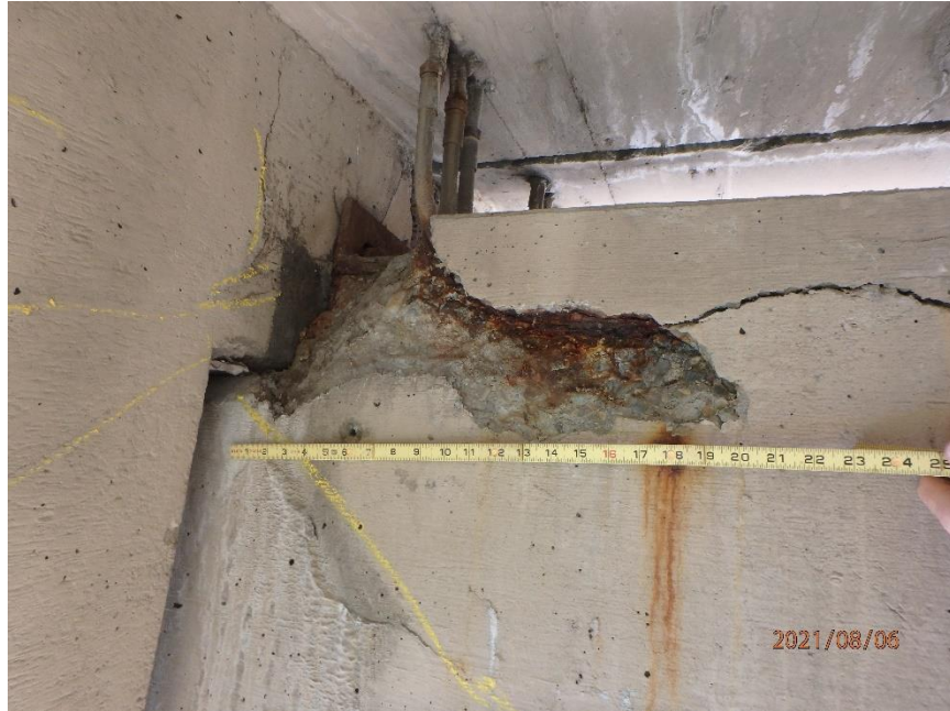
Photo 55: Spall in West Top Corner of Pier 1 Cap South Face, Looking North
