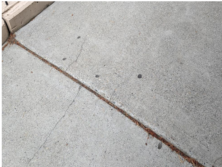
Photo 16: Typical Longitudinal Cracking from Deck Joints in Top of Deck, Looking Southeast
