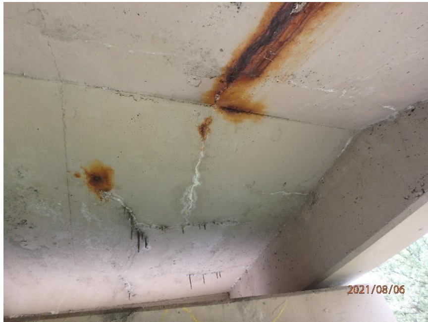
Photo 90: Typical Cracking and Rust Staining in Underdeck, Looking South
