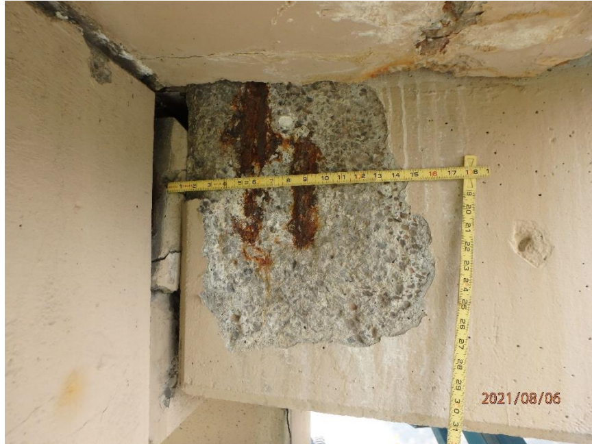
Photo 41: Spall in Span 2 West Girder on the West Face at the North End, Looking East
