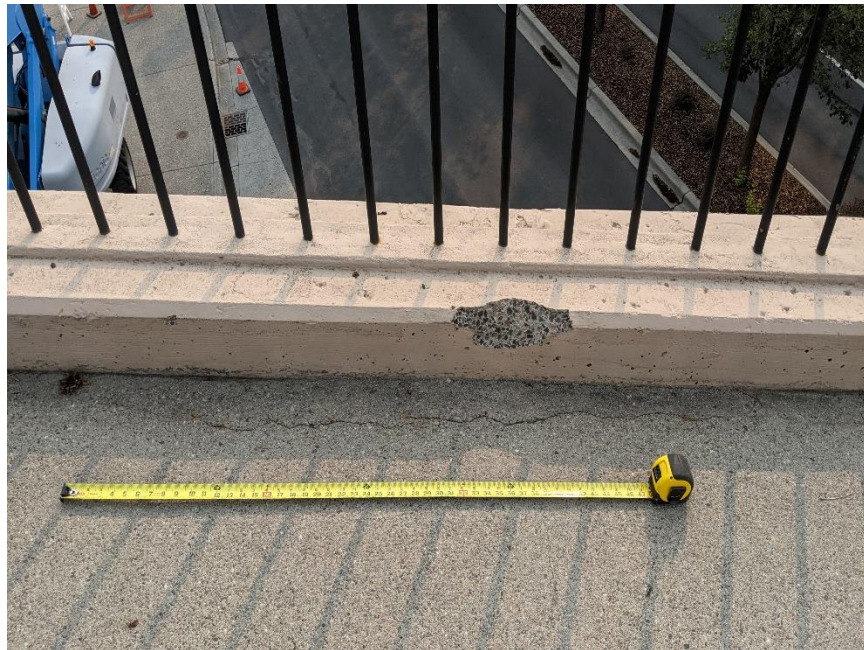
Photo 82: Typical Spalls in Concrete Curb
