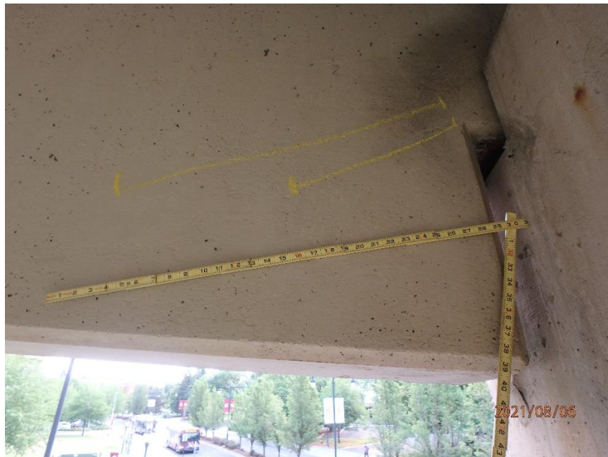
Photo 44: Diagonal Cracks in West Face of Span 3 East Girder at South End, Looking East
