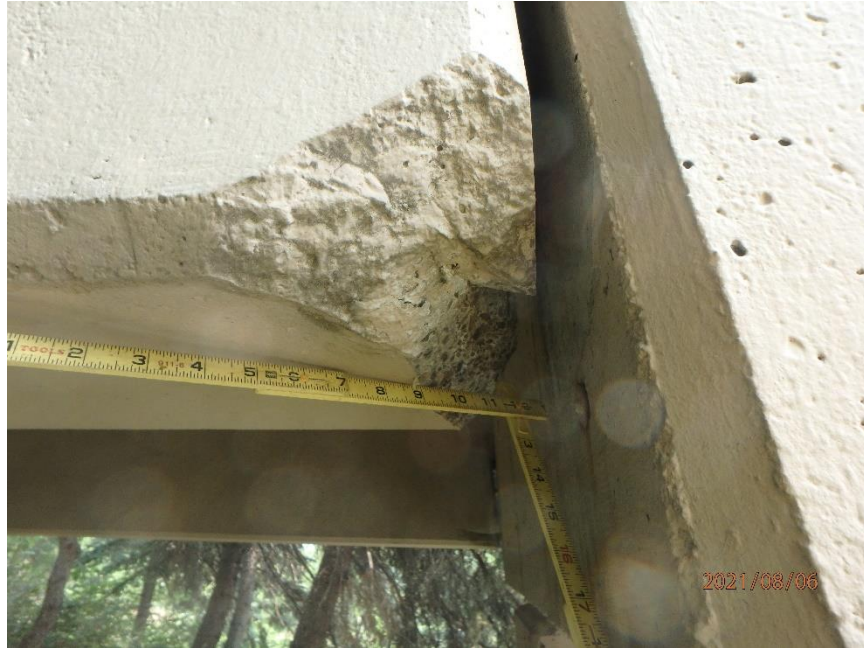
Photo 49: Spall in Span 4 West Girder on the West Face at the South End, Looking East
