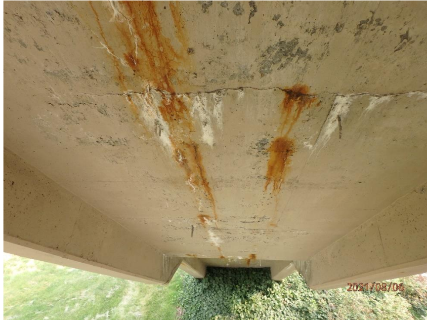
Photo 89: Typical Cracking and Staining in Underdeck, Looking North
