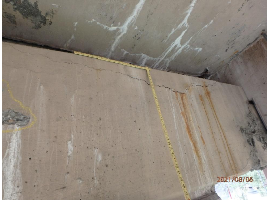
Photo 65: Delamination of the North Face of Pier 2 Cap, Looking Southwest
