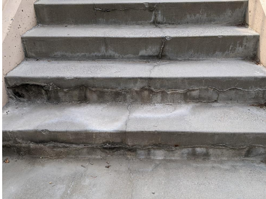
Photo 87: Typical Transverse Cracks and Accumulation in Risers, Looking South
