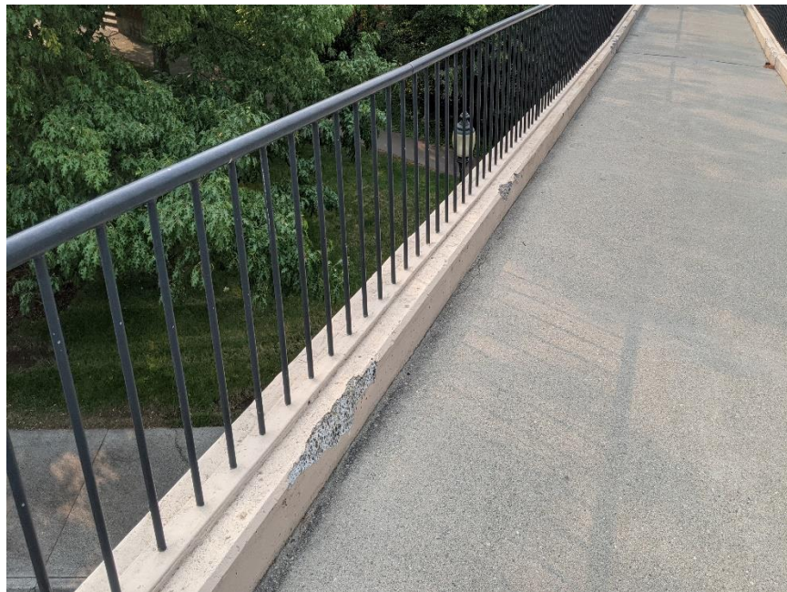
Photo 80: Typical Spalls in Concrete Curb
