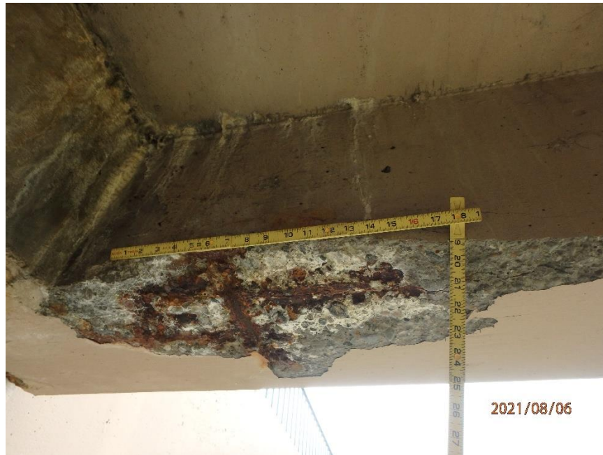
Photo 95: Spall in North Bottom Edge of South Stair Girder, Looking South
