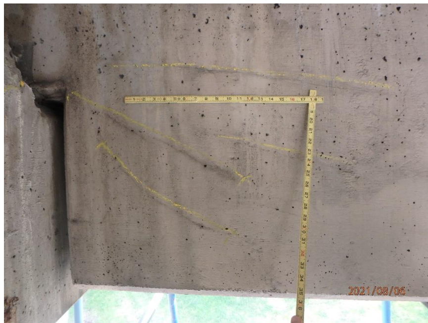
Photo 26: Diagonal Cracks in West Face of Span 1 East Girder at North End, Looking East
