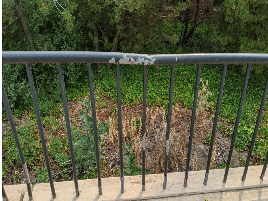
Photo 79: Typical Minor Impact Damage and Chipped Paint in Metal Rail with Typical Rust at Base.
