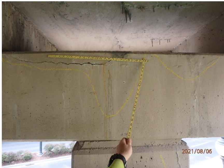
Photo 92: Delamination and Cracking of the North Face of Pier 2B Cap Top Corner, Looking South
