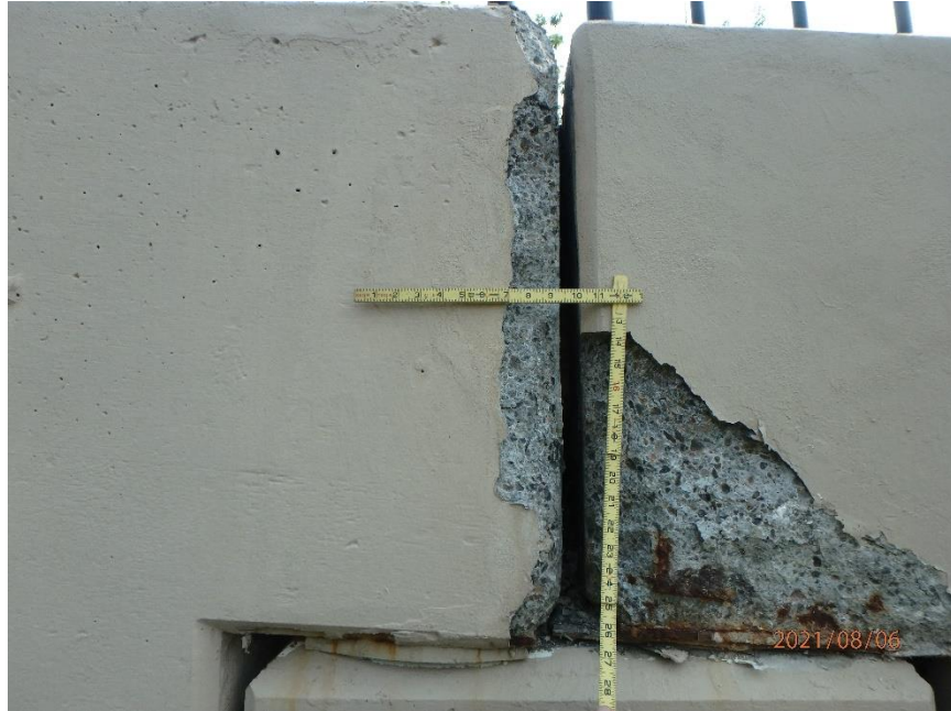
Photo 33: Spall in West Face of Span 2 West Girder at bottom edge at South End. Looking East
