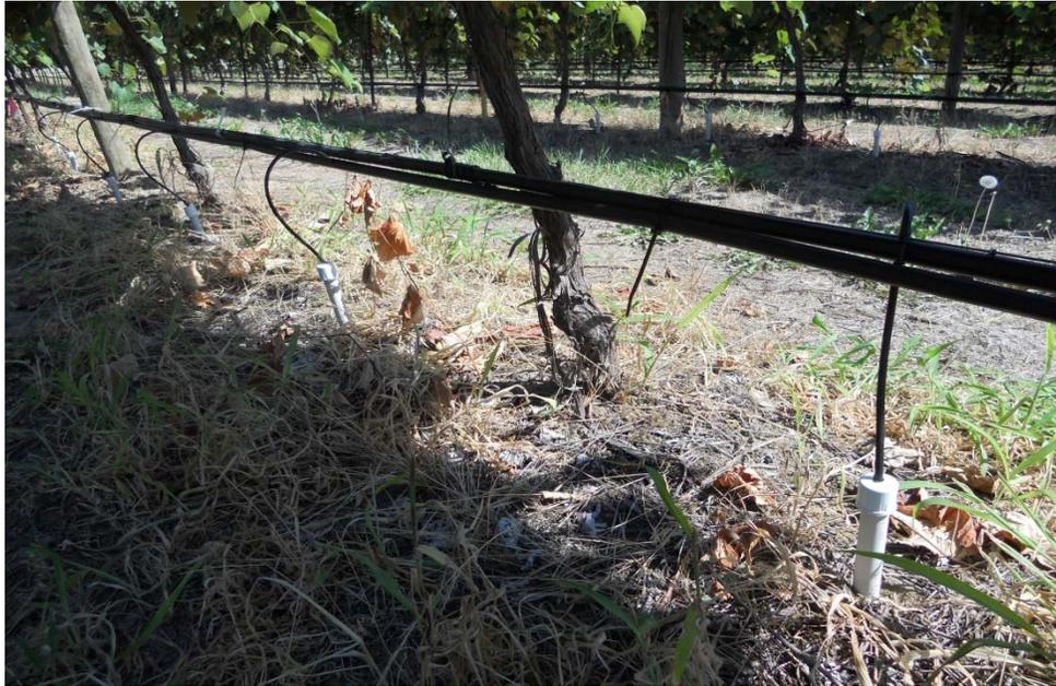
Figure 1. Vertical delivery device containing pressure compensating drip emitter just beneath cap on top of PVC tube.
