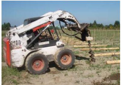
Figure 1. Drilling postholes for end posts
