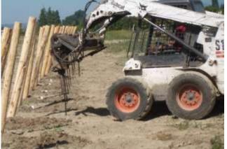
Figure 8. Drilling in post anchors
