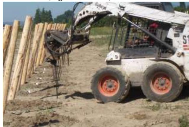
Figure 8. Drilling in post anchors
