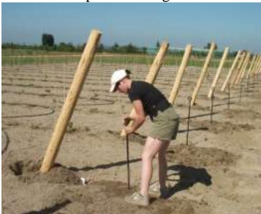
Figure 7. Setting post anchors
