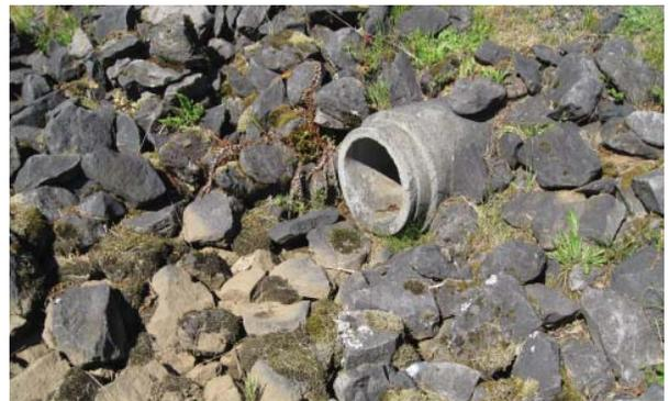
*Stormwater outflows often have a layer of rock preventing erosion as water flows out after storms.*
