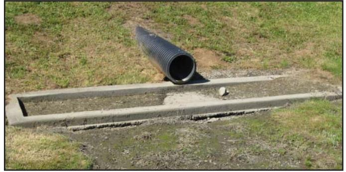
*A level spreader. Inspect for sinkage, damage or erosion.*
