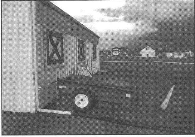
Runoff from the barn roof is directed away from the barn and turnouts using gutters, downspouts and inexpensive pipe extensions. The new manure spreader is used to spread finished manure onto pastures.
