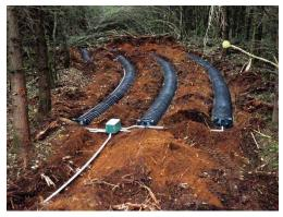
Your drainfield is critical to the health of your septic system and needs to be protected. The pipes and other components in your system may not be buried very deep below ground and could be easily crushed. The soils in your drainfield contain oxygen-loving bacteria that break down and filter the effluent. If the area is compacted by driving or parking on it, the bacteria won't be as effective and will reduce the ability of the water to percolate
