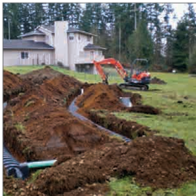
Drainfield installation (Photos: Alan Chapin)
