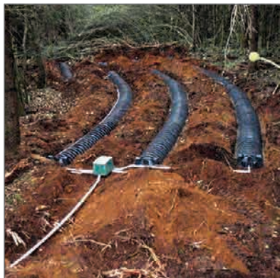
Drainfield installation (Photos: Alan Chapin)
