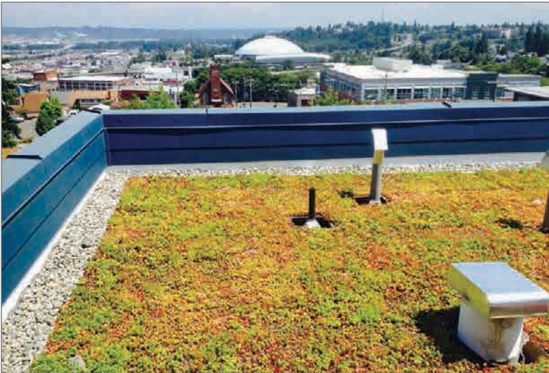
Green roof (Photo: Solterra Systems)
