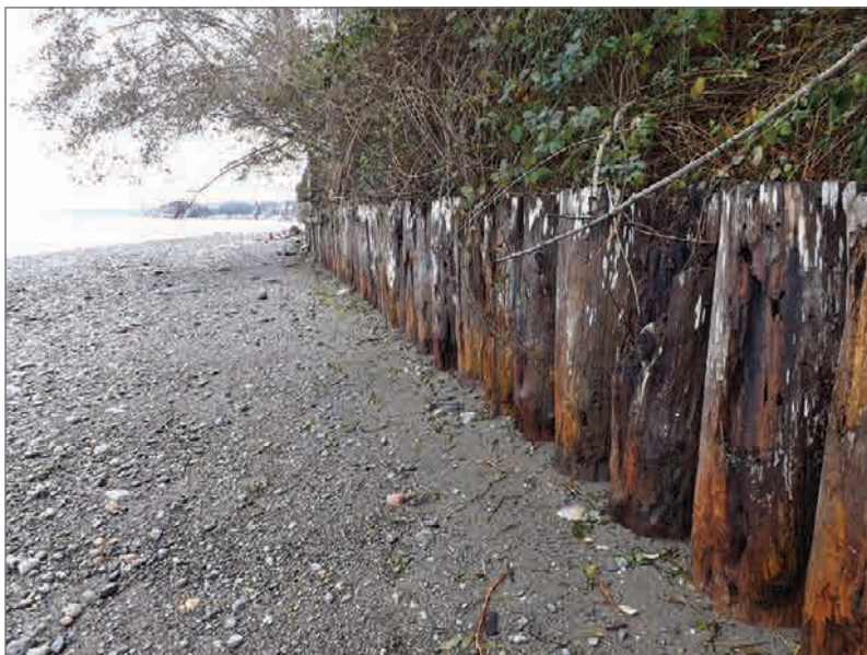
Eroding wood bulkhead (Photo: Scott Chase)
