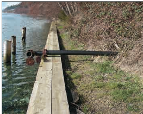
Tightline dissipater (Photo: Scott Chase)
