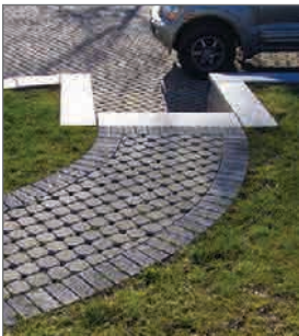
Left: Permeable pavers (Photo: Interlocking Concrete Paving Institute) Right: Porous concrete (Photo: Kathleen Chase)
